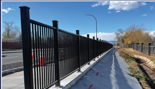
NEW RAILING AT NOBLES TRIBUTARY
