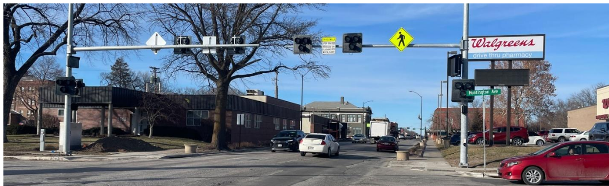
Pedestrian Hybrid Beacon, a Proven Safety Countermeasure.
