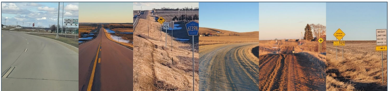
TRIPP COUNTY ROADWAY SURFACES VARY FROM CONCRETE PAVEMENT TO UNPAVED GUMBO (PIERRE SHALE) ROADS IN THE NORTH AND CLAY ROADS IN THE SOUTH. SOURCE: FHU 2024
