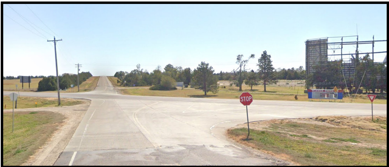
Skewed intersections cross US 18 and SD 44 on 317 th Ave east of Winner. Source: Google Streetview
